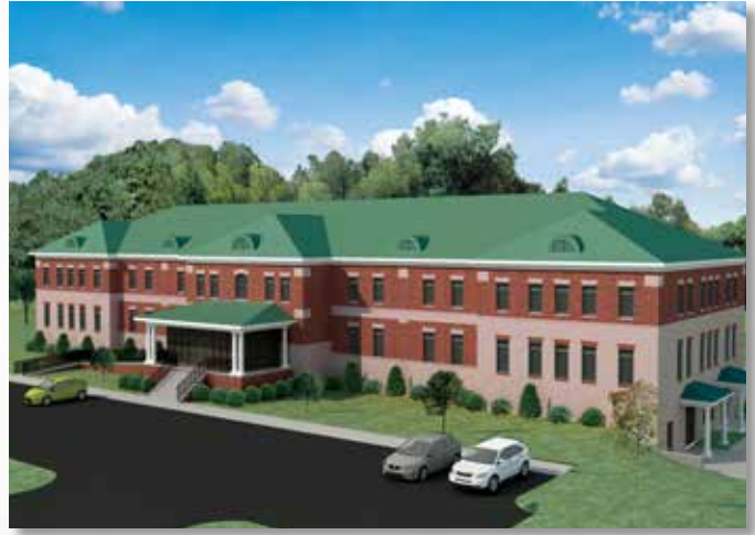
The Pruitt Family Behavioral Health & Administration Center is currently under construction and will be completed by the end of 2022.
